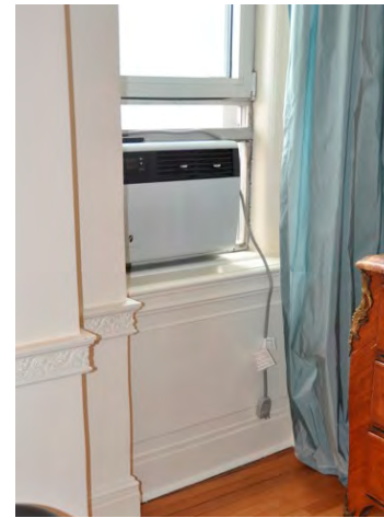
DINING ROOM -Plexi-glass seal around AC unit
