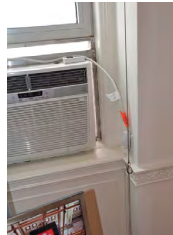
RECEPTION ROOM -Plexi-glass seal around AC unit
